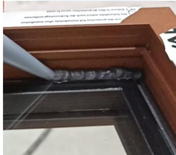
4. Fill the remaining space using structural glue on glass circumference.
